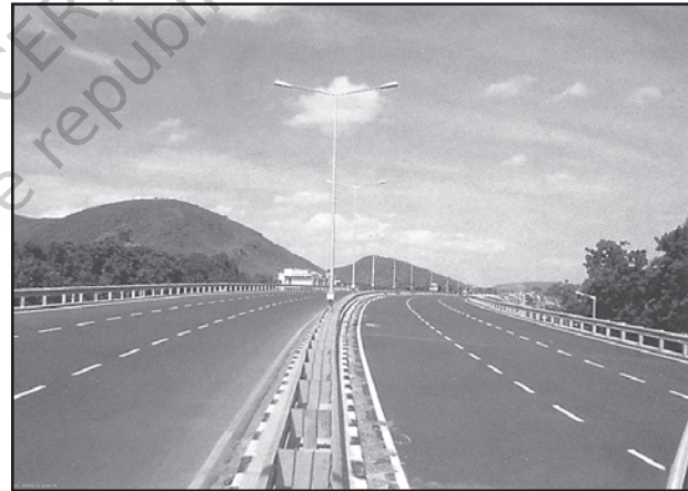
Fig. 8.3 : Dharmavaram Tuni National Highway, India
